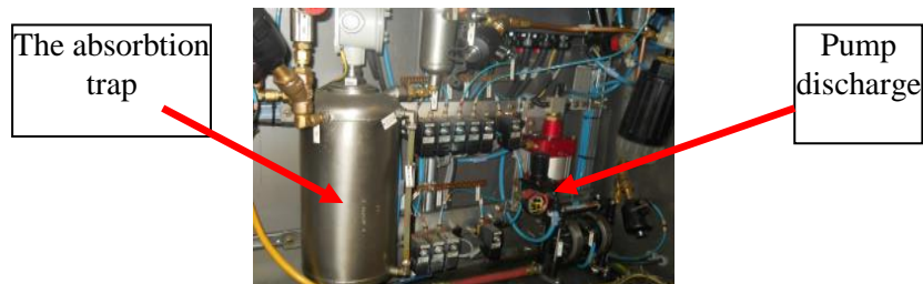
Figure 1. The installation of priming
